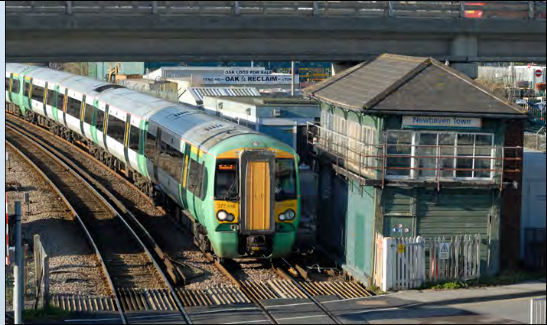
Right: Southern Railway's Class 377 448 arrives at Newhaven Town, East Sussex on the 2F81 Brighton - Seaford service, March 22nd. The signal box was built in 1879, in 1953 it received a brick extension at the rear to allow the installation of a larger lever frame that was previously used at Three Bridges. The building looks as if it does need the support of the extension. However the box could close in 2015 with control passing to the Sussex Regional Operations Centre at Three Bridges. Gary S. Smith
