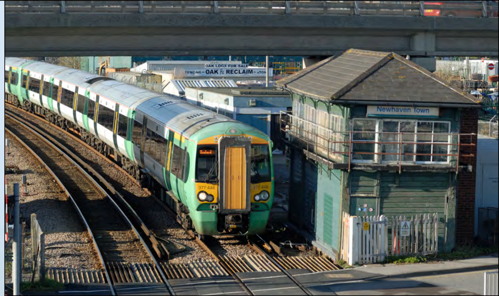
Right: Southern Railway's Class 377 448 arrives at Newhaven Town, East Sussex on the 2F81 Brighton - Seaford service, March 22nd. The signal box was built in 1879, in 1953 it received a brick extension at the rear to allow the installation of a larger lever frame that was previously used at Three Bridges. The building looks as if it does need the support of the extension. However the box could close in 2015 with control passing to the Sussex Regional Operations Centre at Three Bridges. Gary S. Smith
