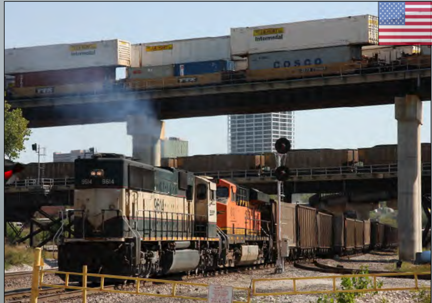
Right: Full house at Kansas City Bottoms. Double stacks pass each other on the BNSF flyover, beneath it a Union Pacific coal loads heads over the Union Pacific flyover having just crossed the Kansas River on the upper deck of the Adams Street Bridge. On the ground a BNSF coal working rattles over the diamonds with another 2 BNSF locos on the rear assisting. Andy Pratt
