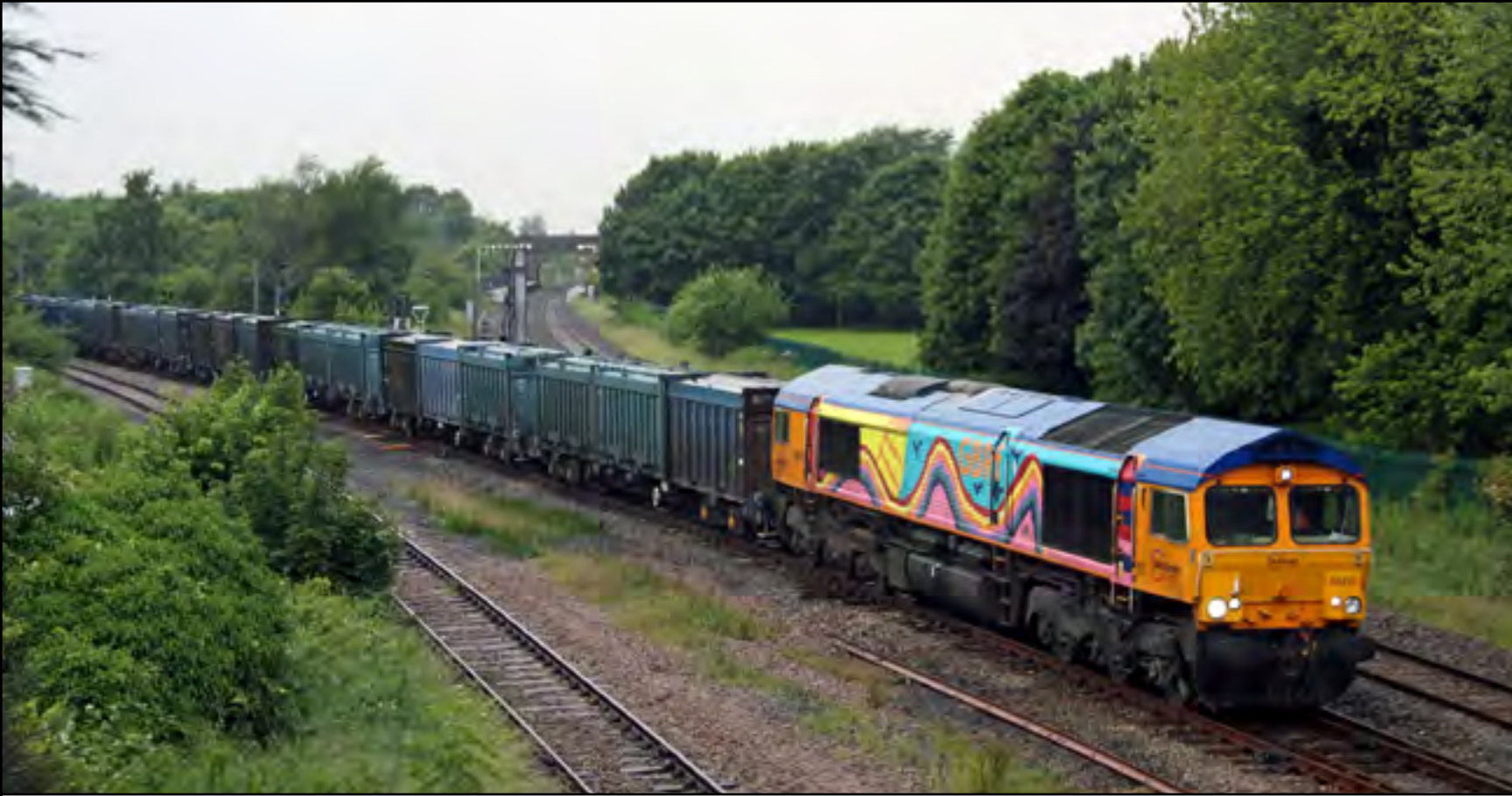
Above: Class 66 720 hauls the 4C77 Fiddlers Ferry power station to New Biggin (Gbrf) through Lostock Junction on July 2nd. Alan Naylor
