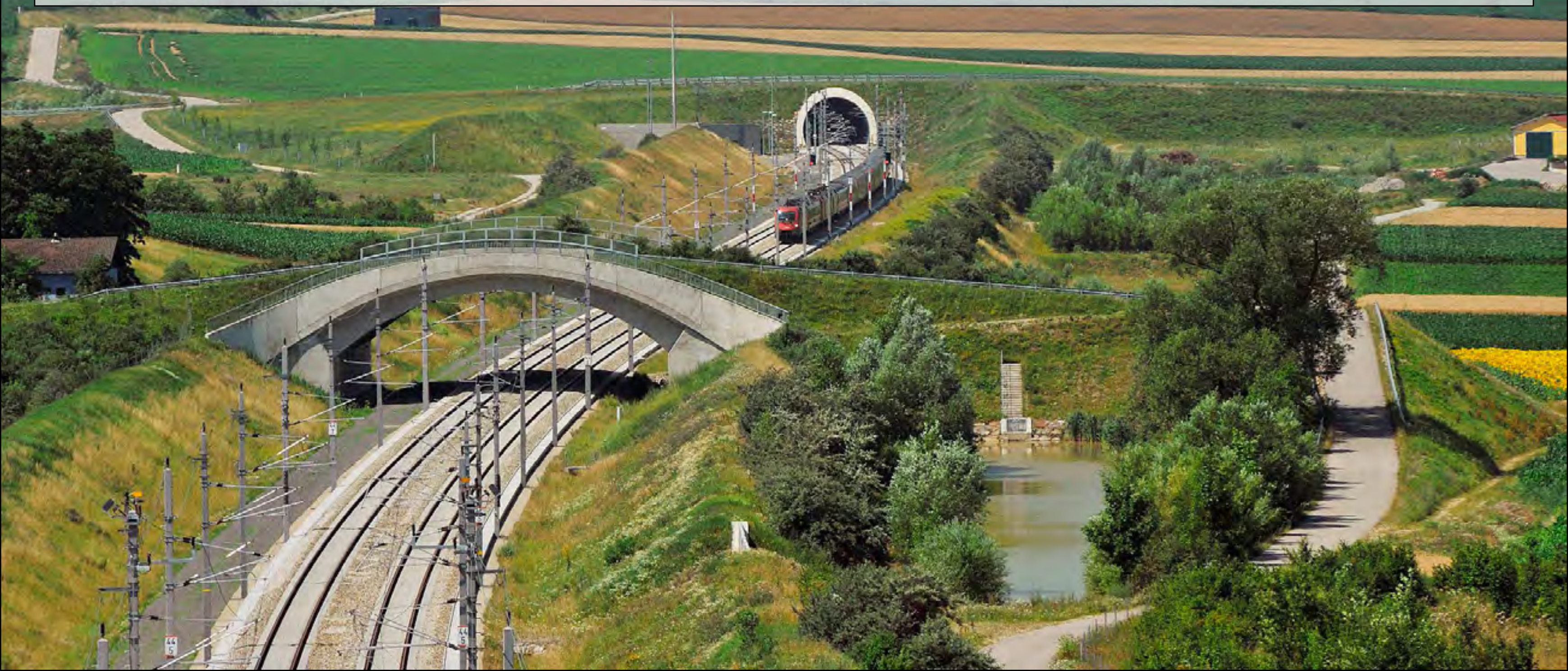
Photo: Robert Deopito - The New high-speed route between Wien and St. Polten.
