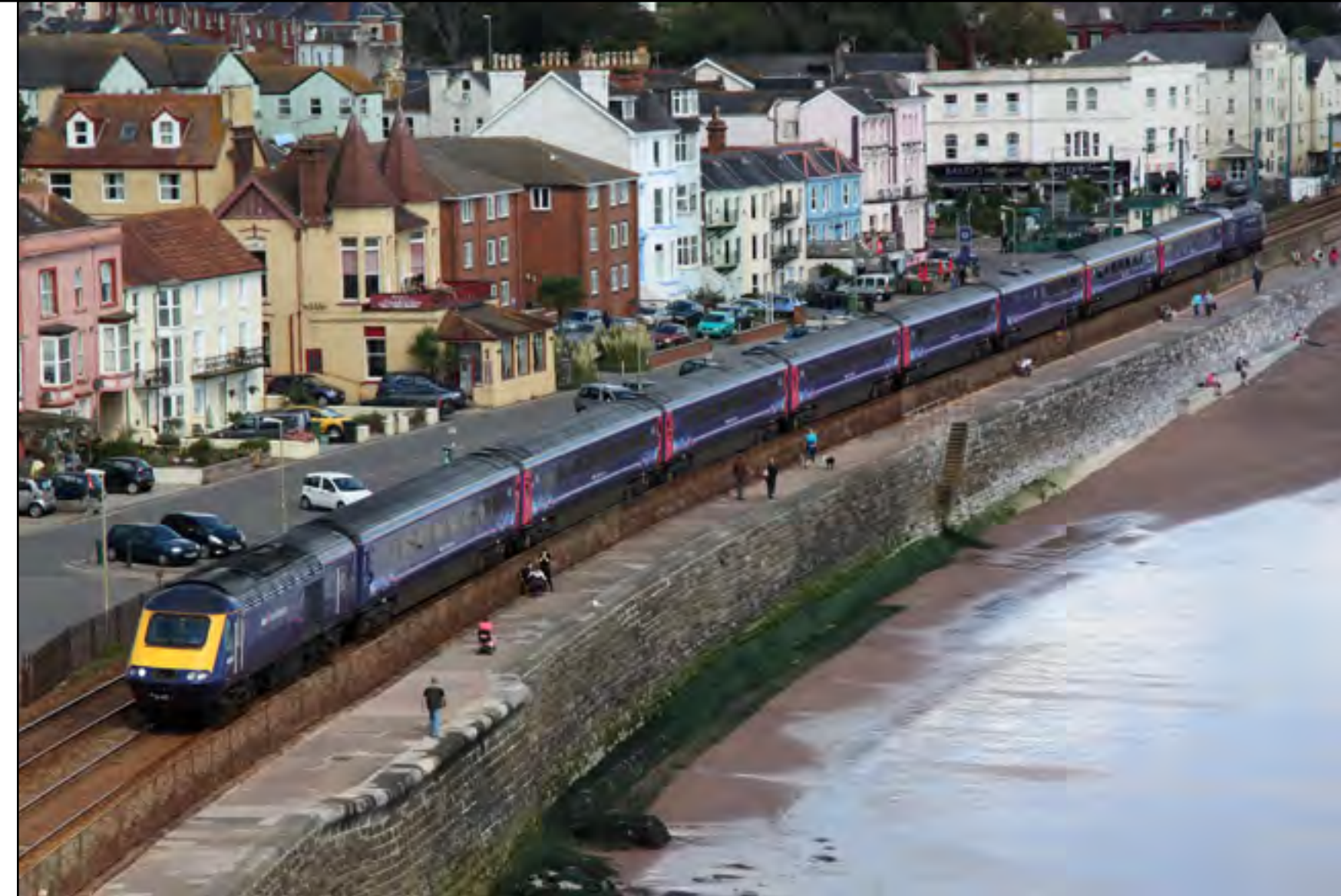
Top Right: On September 18th, FGW HST power car No. 43162 heads a London Paddington - Penzance service along the sea wall at Dawlish. Phil Martin
