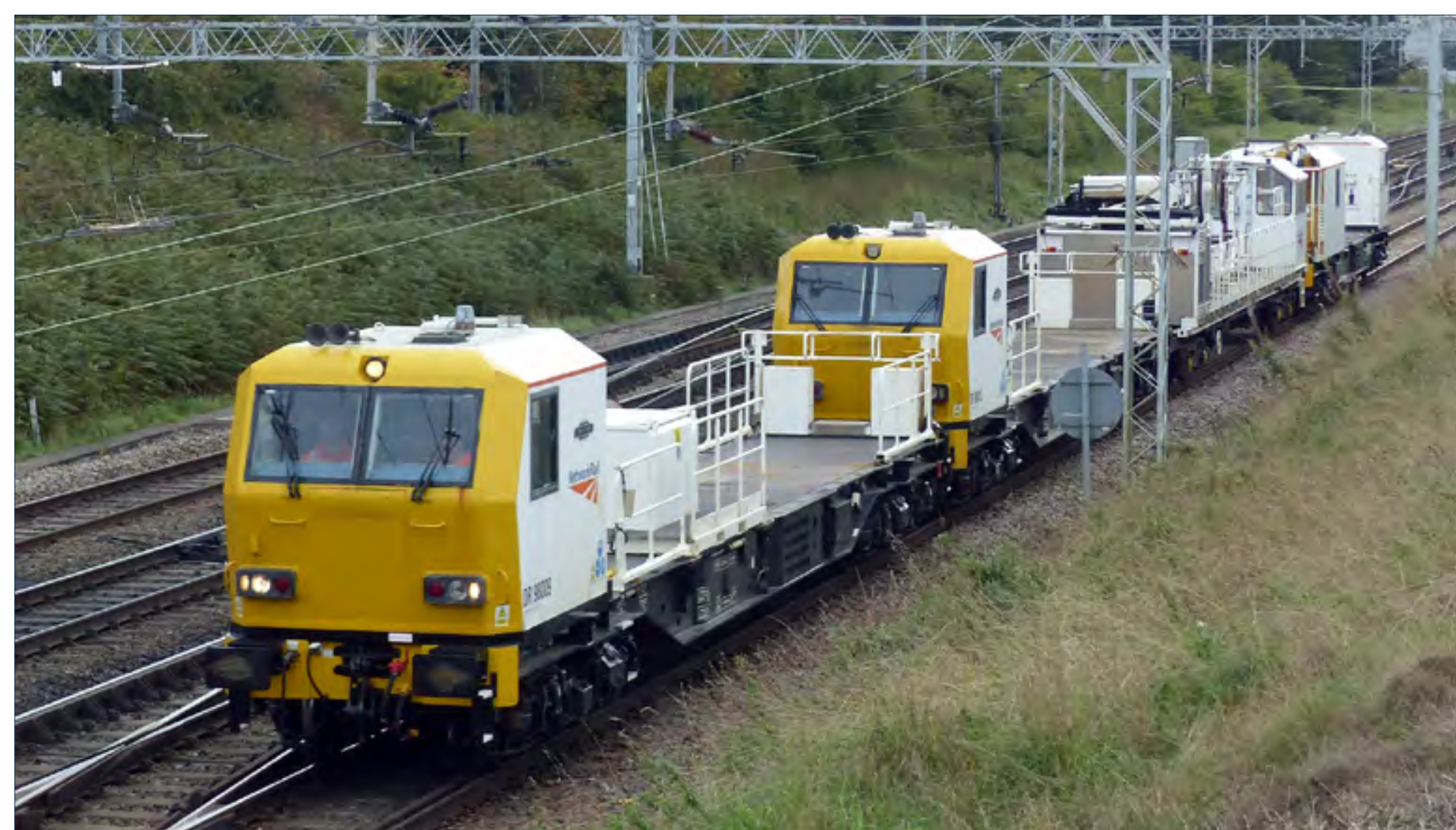
On September 22nd, track repair and maintenance machines Nos. DR 90809, 90812 and 90814 approach Basford Hall Yard working from Bescot - Crewe Electric Depot. Michael Lynam
