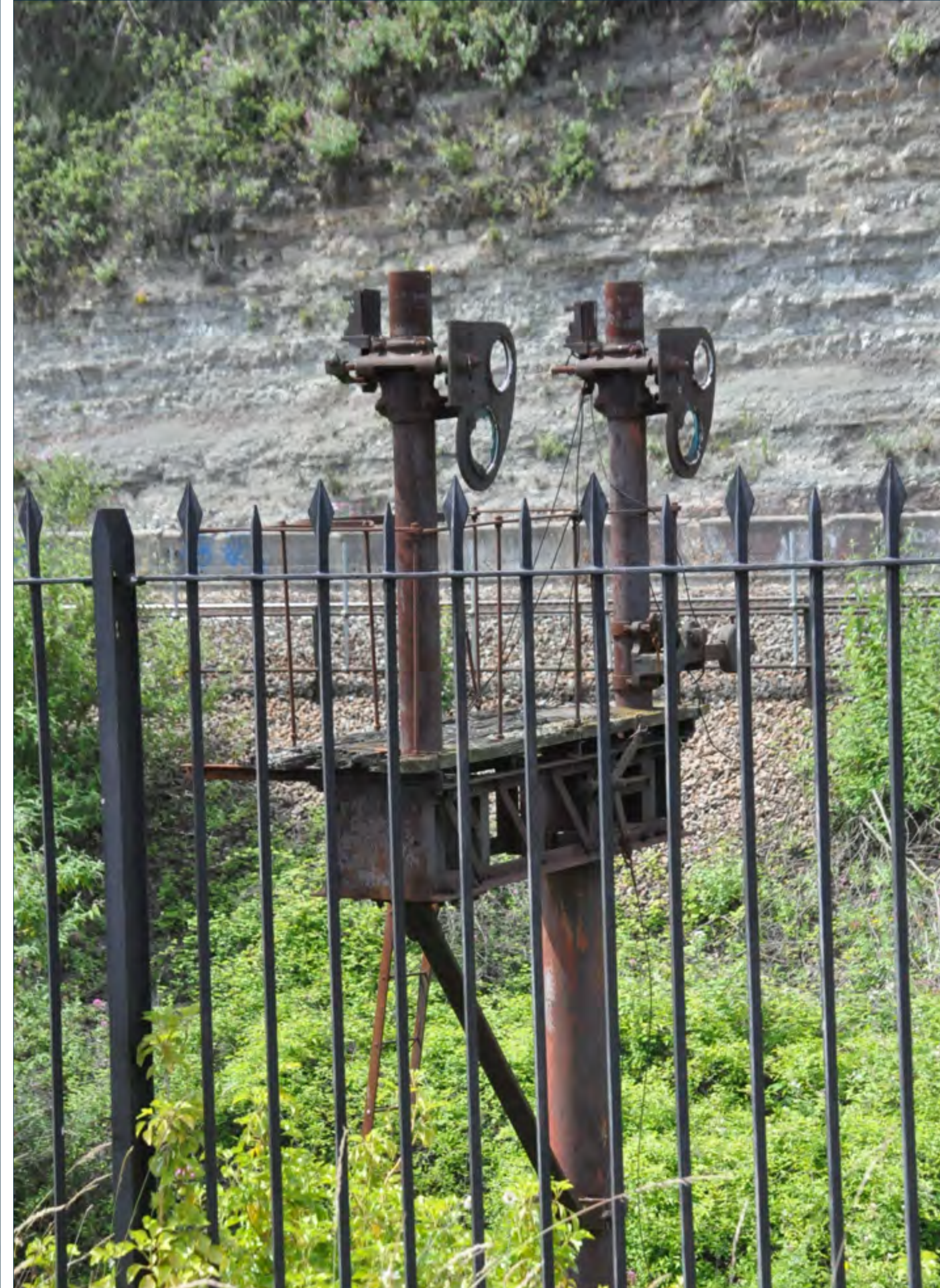
Old signals on the Cadaxton to Barry line about a mile east of Barry Station. Ken Mumford
