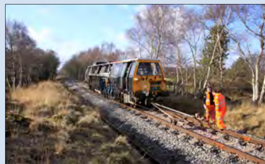
Furzebrook to Creech Bottom track tamping, carried out on March 5th.
