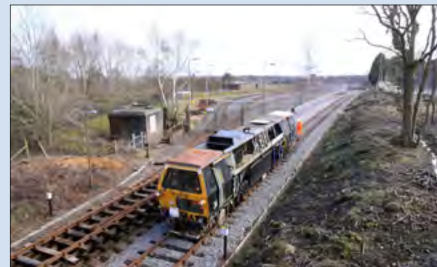
Furzebrook to Creech Bottom track tamping on March 5th.
